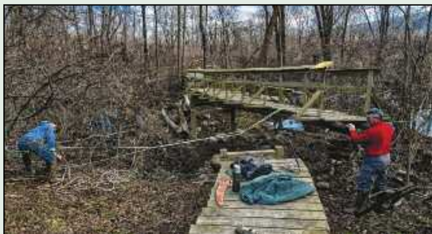
West Jersey Crew members move a bridge segment back into place.
